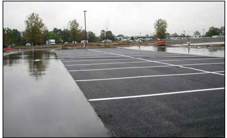
Permeable pavement. Source: EPA
