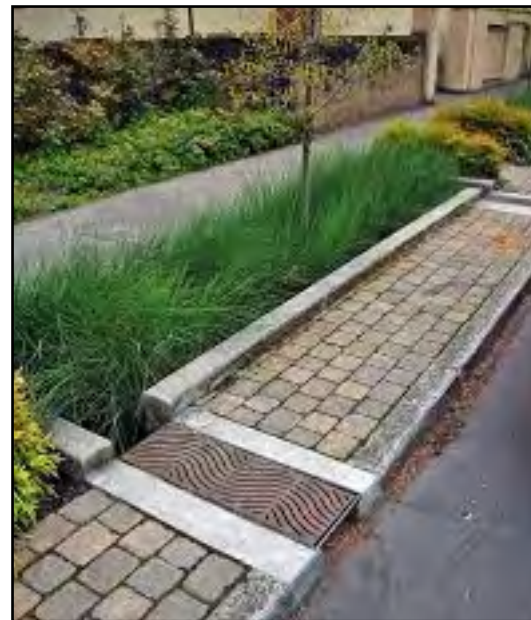
Roadside bioretention. Source: sitephocus.com
