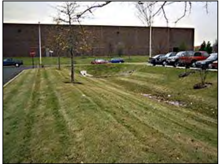
Grassed swale. Photo Source: EPA
