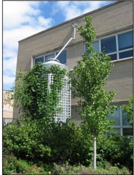
Distributed Site Design Measures, such as this cistern, can provide significant reductions in site runoff.
