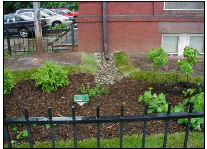
Rooftop disconnection. Source: LID Center
